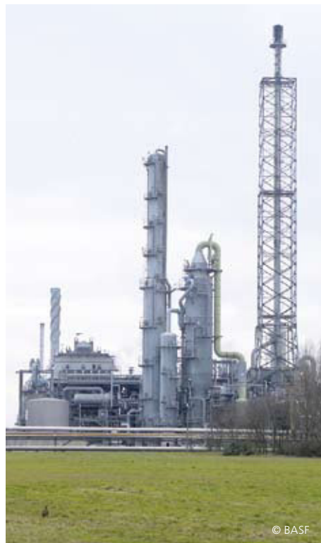
Ammonia production plant of the company BASF
